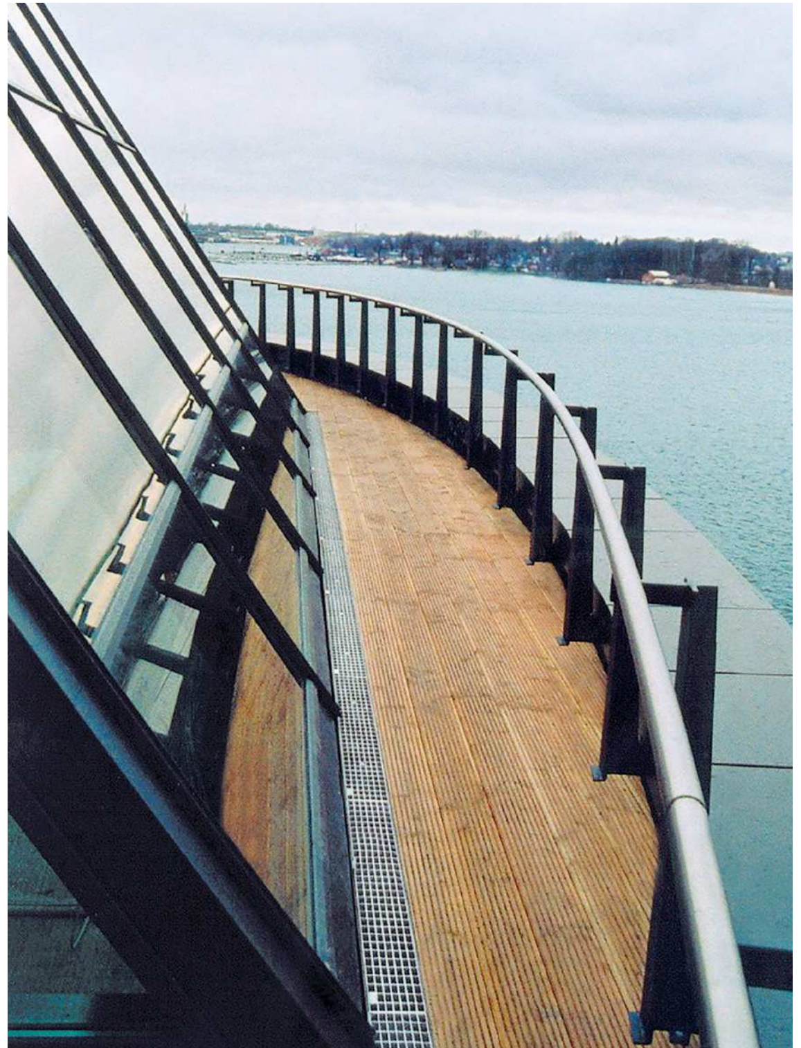
SILO4 Rostock, Germany ■ FACADE DRAINAGE
